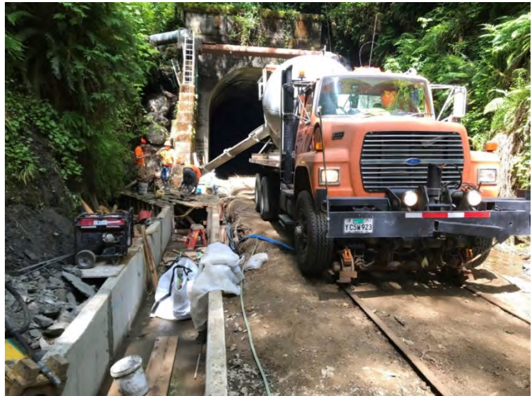
Photo: Concrete work at Tunnel 19.
