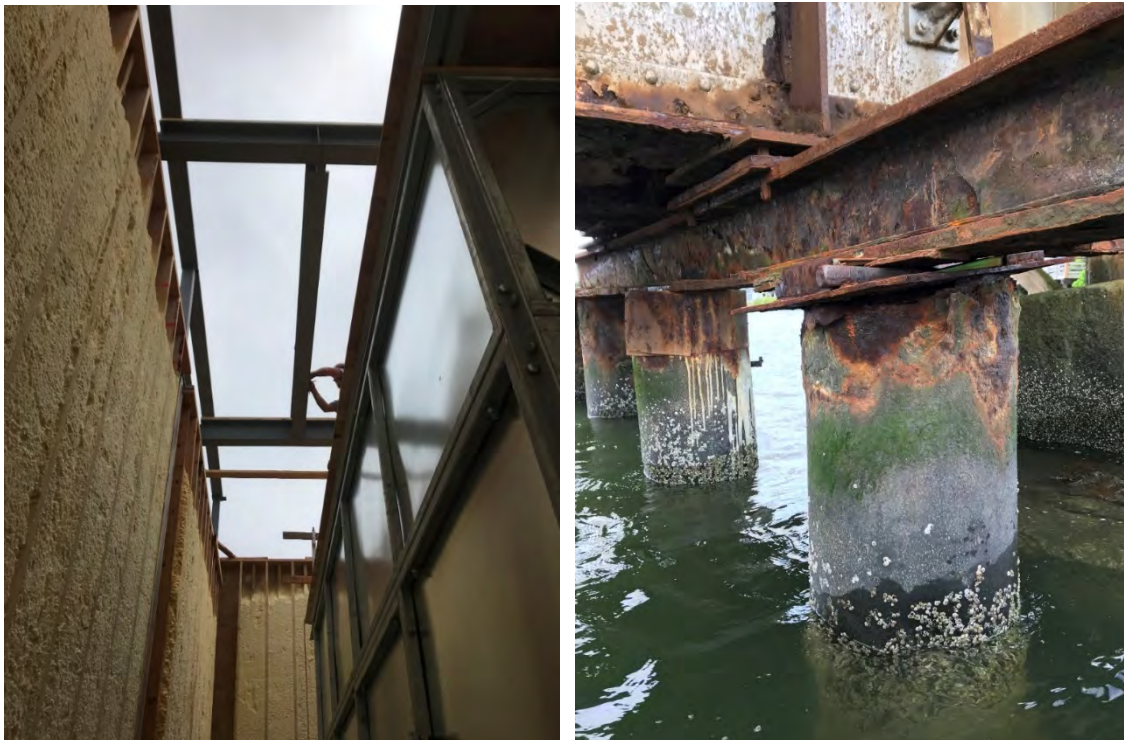
Photos: Ice Plant construction (left). Coalbank Slough Bridge (right).
