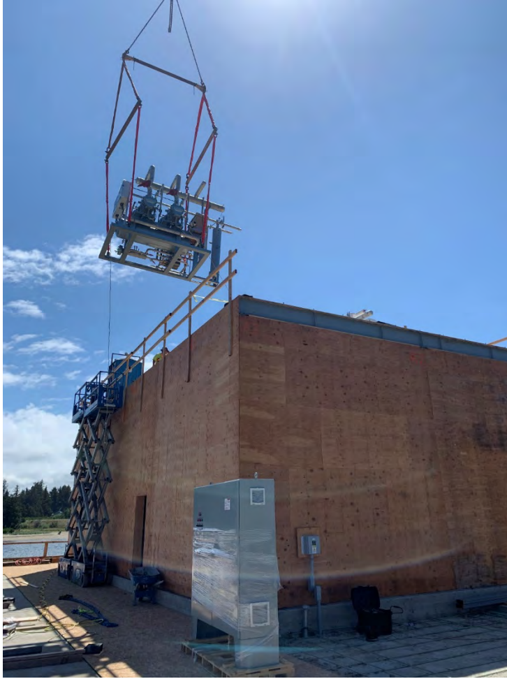
Photos: Compressor skid lift on Wednesday, July 1 (left). Twin 90 ice makers mounted on Thursday, July 2 (right). Bin wall construction on Thursday, July 2 (below).
