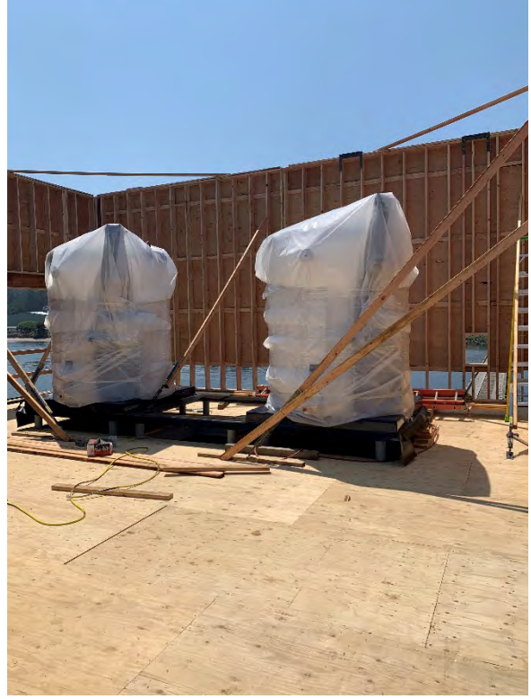
Photos: Compressor skid lift on Wednesday, July 1 (left). Twin 90 ice makers mounted on Thursday, July 2 (right). Bin wall construction on Thursday, July 2 (below).
