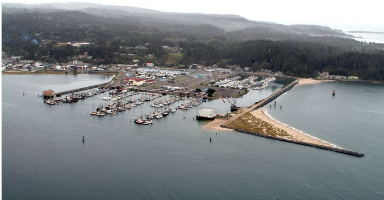
Figure 2-17: Charleston Marina and Breakwater, Looking West
