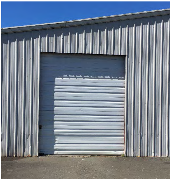
Photo: Wider overhead door installed for vehicle access.
