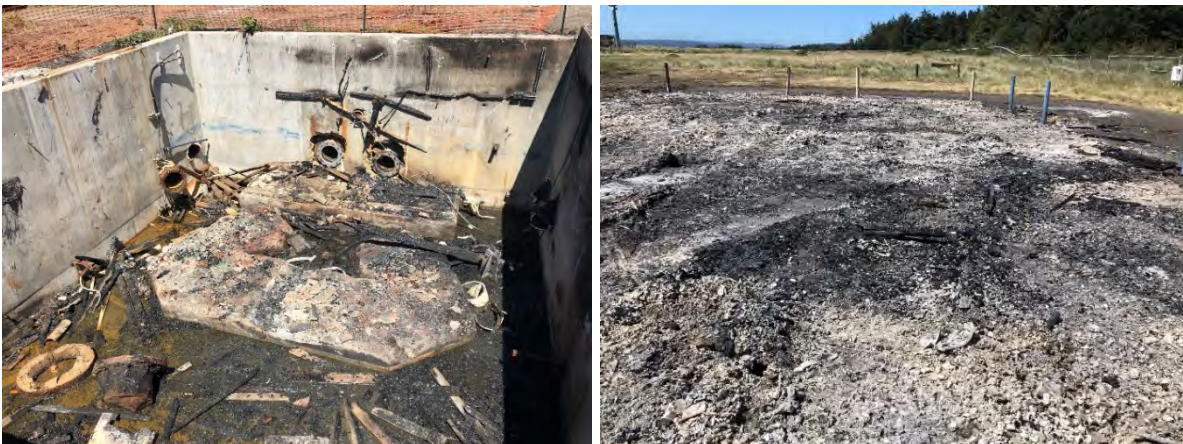
Photos: Pit from Fish Farm water pump station (left), and Remains of Fish Farm Admin Building (right).
