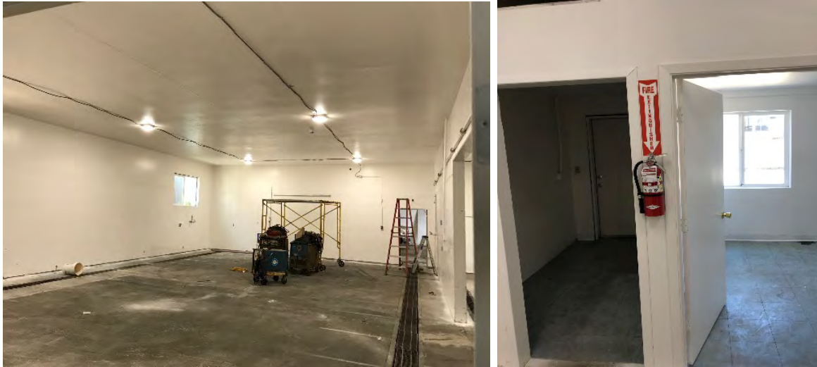
Photos: New LED lighting and Safety Equipment.
