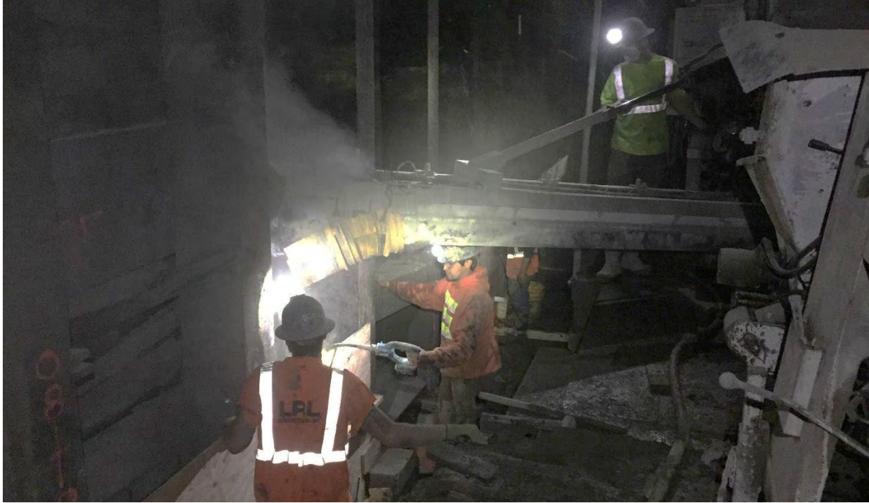
Photo: Tunnel 13, Pouring concrete into the formed set.
