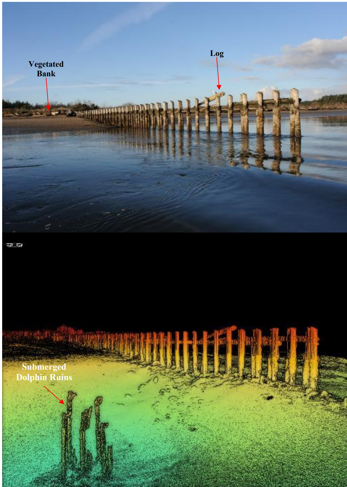
Figure 34. Pile Dike 7.3 viewed from downstream looking shoreward.
