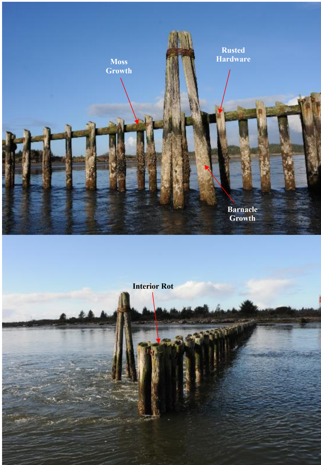
Figure 30. Pile Dike 7.0 photographs of the pile condition and hardware.
