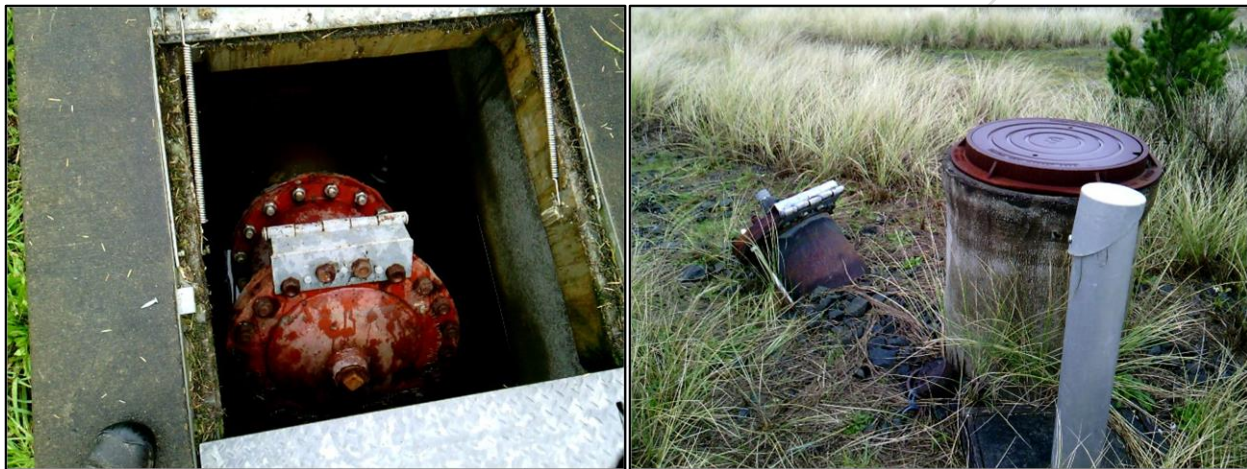
Figure 7: Water-line vault (left); water-line bore exit (right)
