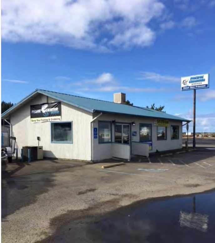
Photo: New Office Building
