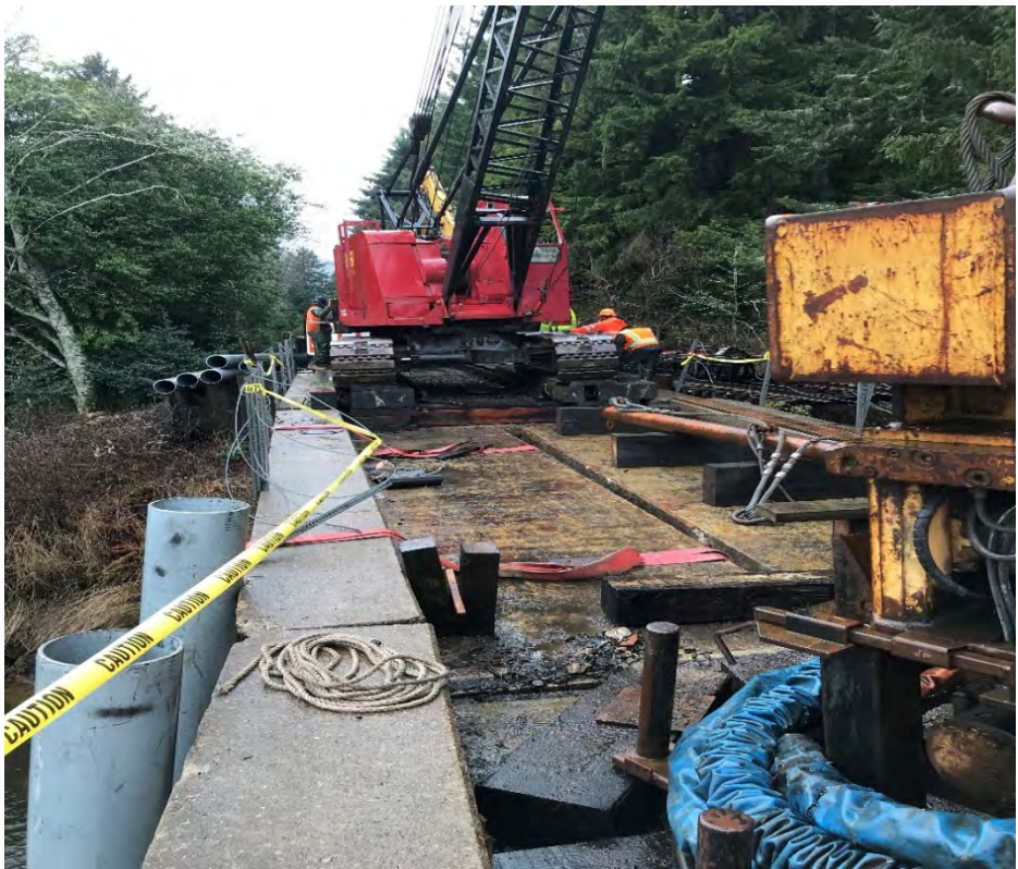
Photos: Scofield Creek MP-740.84 bridge repair work
