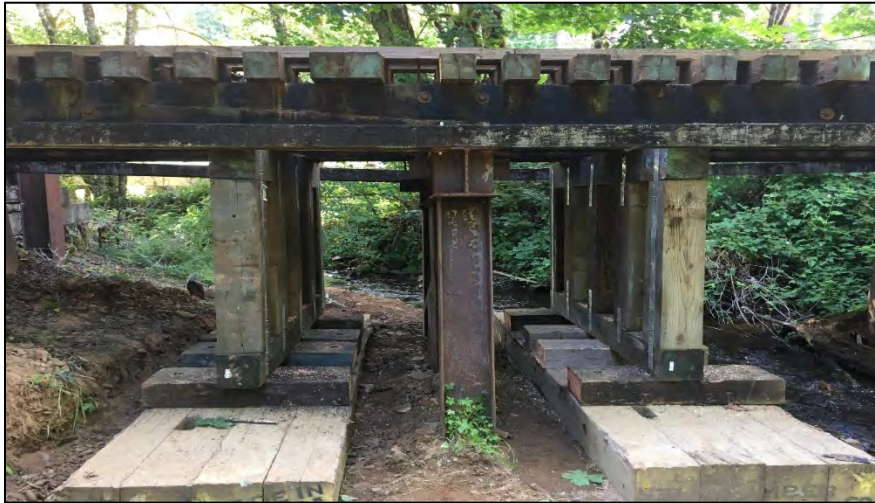
Photo: Walker Creek, Walton, OR MP-677.05 bridge repairs
