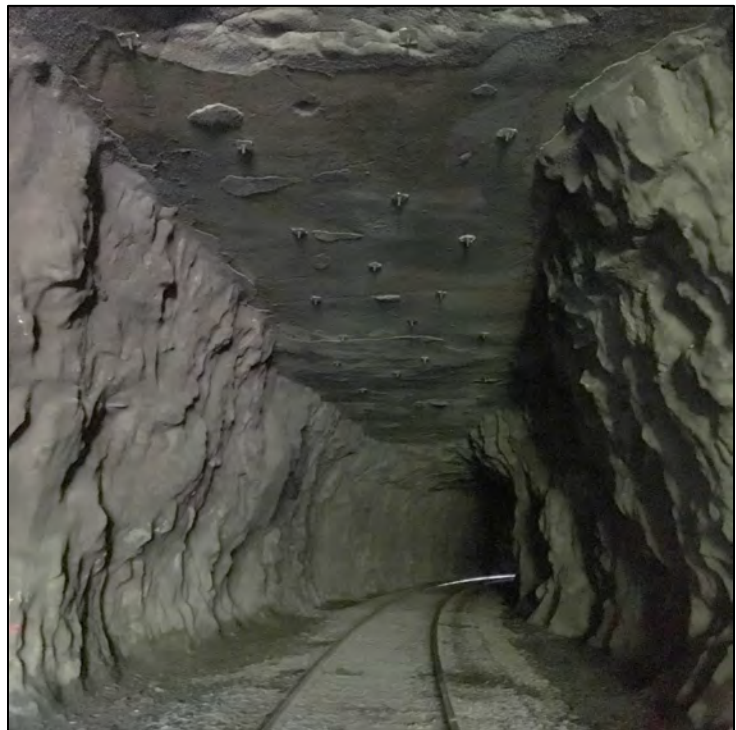
Tunnel 14: Rock bolt installation in tunnel crown
