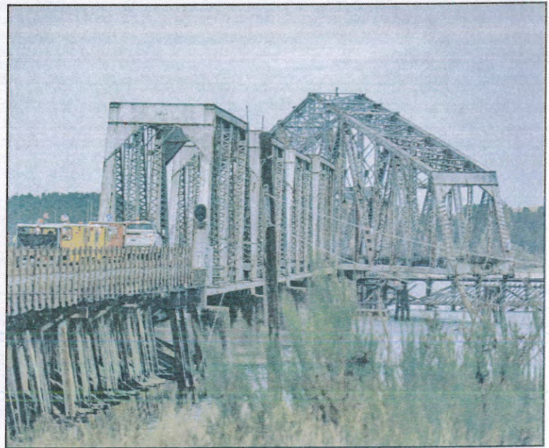
Above right: Rich Gunn operates one of the five Missouri Pacific MT-14M cars at this event. Center left: PRO Treasurer Bob McCoy collects donated toys in his truck. Center Right: The North Bend drawbridge 485-foot swing span closes so we can pass on north to setoff. Below: The front half of the consist stops at the Coos Bay Boardwalk for motorcars to leave toys for distribution by the Rotary club. See Teddy Bear Express story in this issue.
