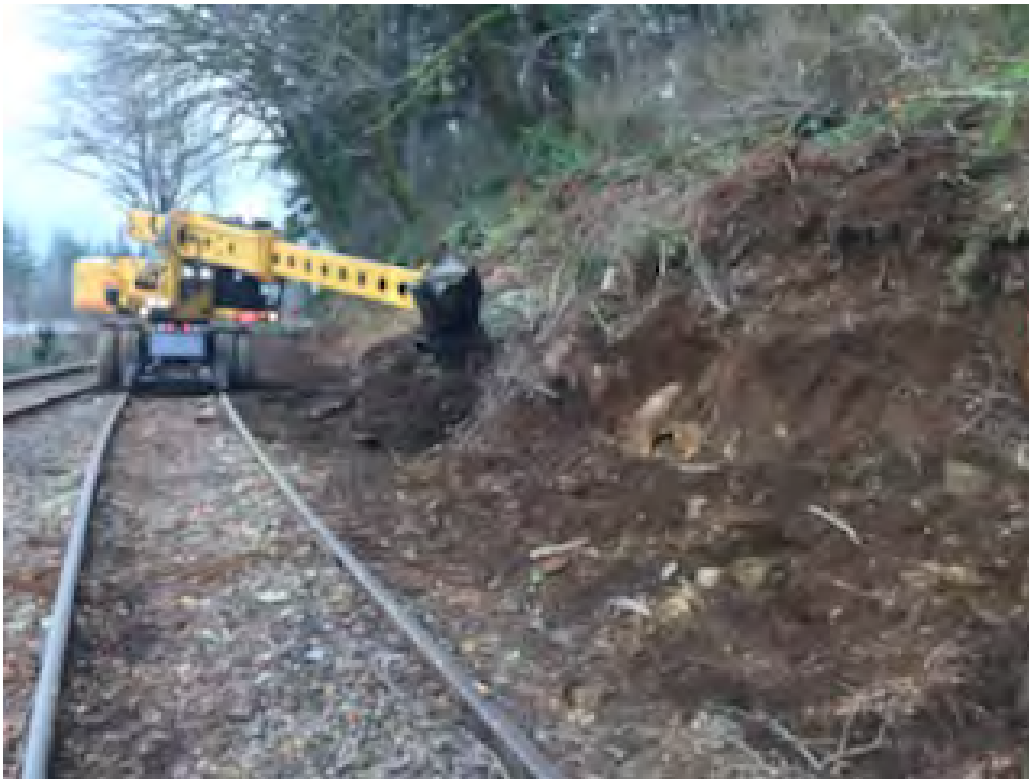
Photo: Gradall working on walkways and ditching at Beck, OR.
