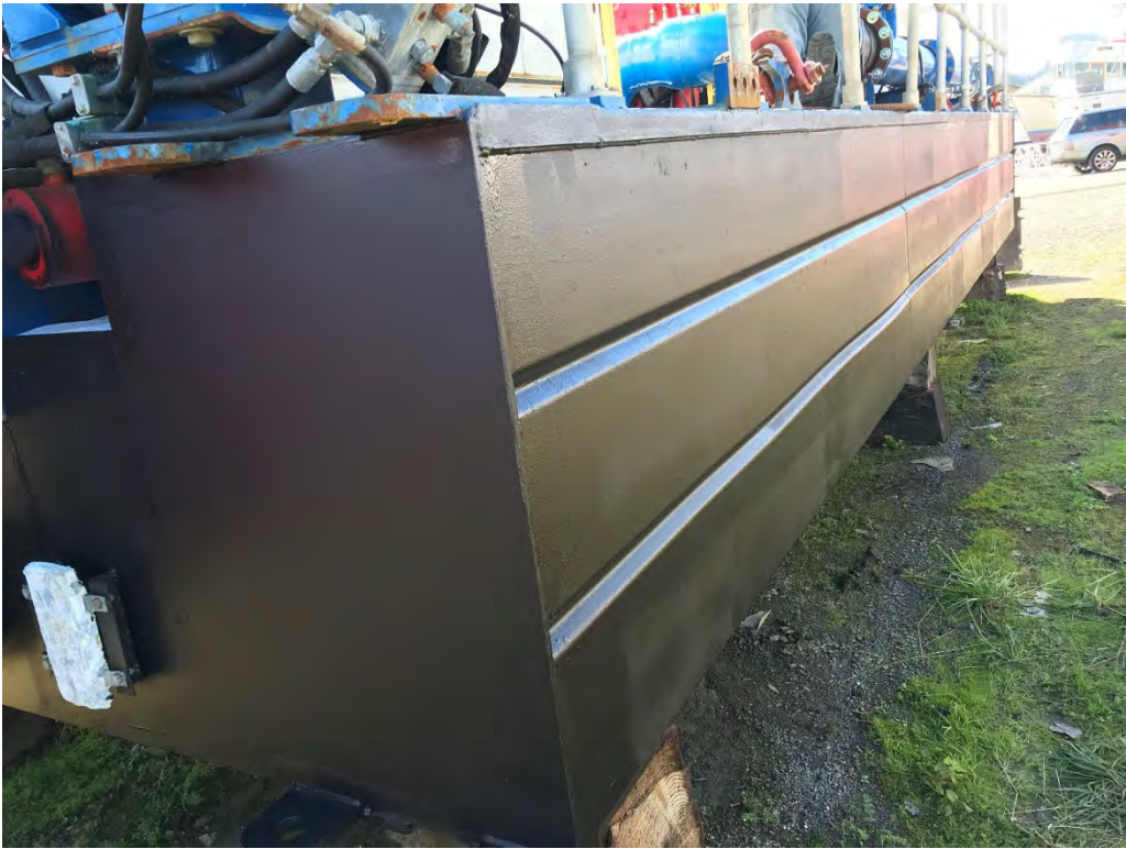
Photos: Dredge Painting
