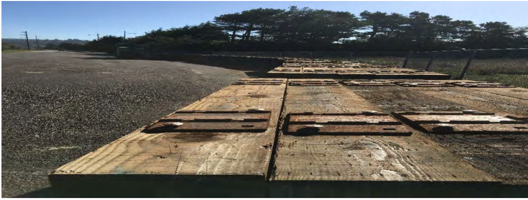
Photo: Staging of pre-plated ties at Jordan Cove transload facility
