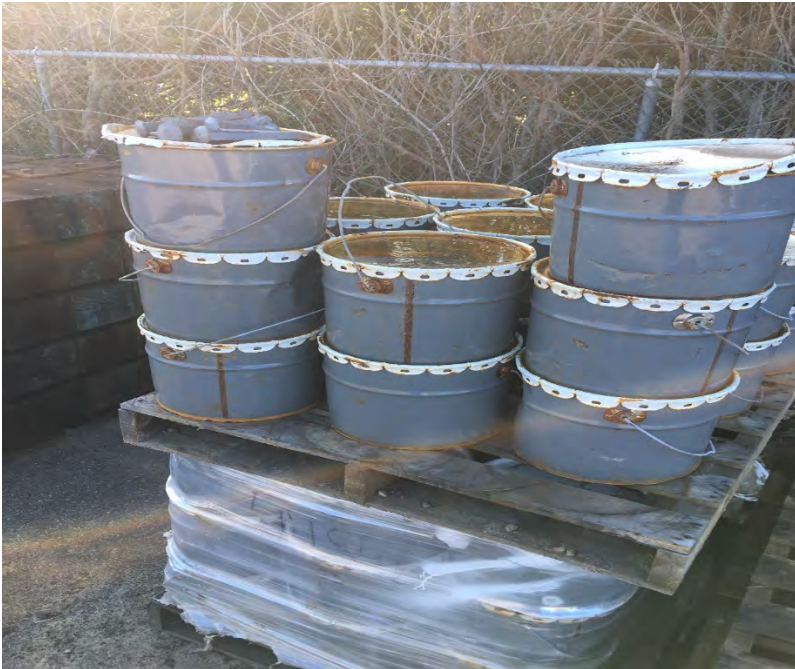
Photo: Staging of new spikes at Jordan Cove transload facility
