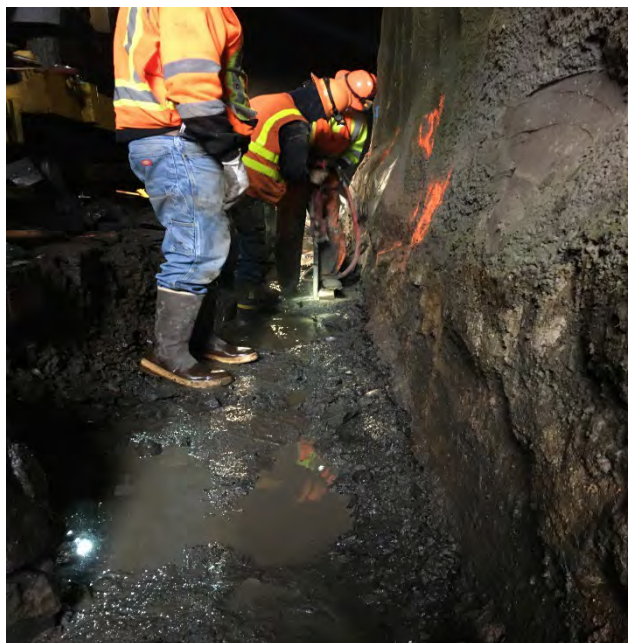
Photos: Crews drilling fracture line in East ditch of tunnel 19 (left). Crews completing saw cutting of East ditch at tunnel 20 (right).
