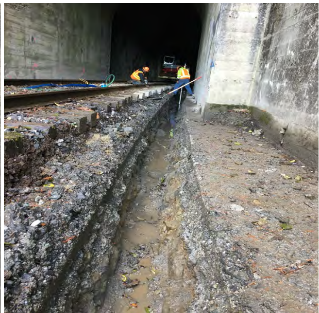
Photos: Crews drilling fracture line in East ditch of tunnel 19 (left). Crews completing saw cutting of East ditch at tunnel 20 (right).
