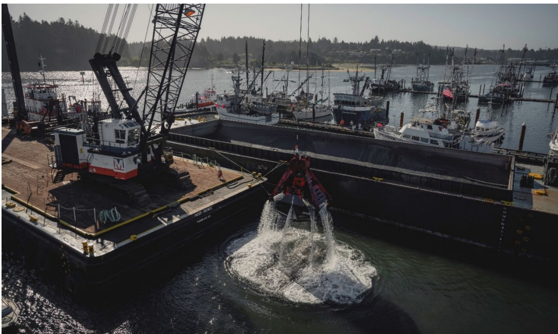
Photo: McAmis dredging 3,000 cubic yards from Point Adams on August 31, 2020.
