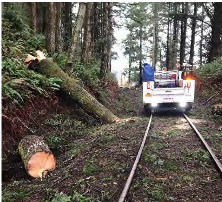
Photos: Hazard Tree Removal by the Maintenance of Way team.
