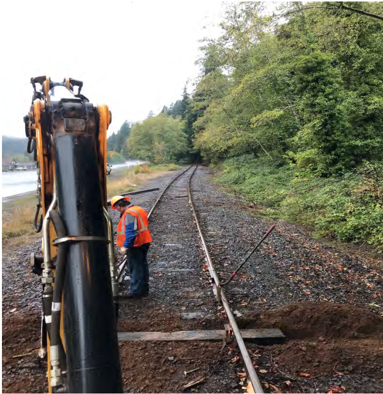
MOW Crew replacing ties at MP 709.
