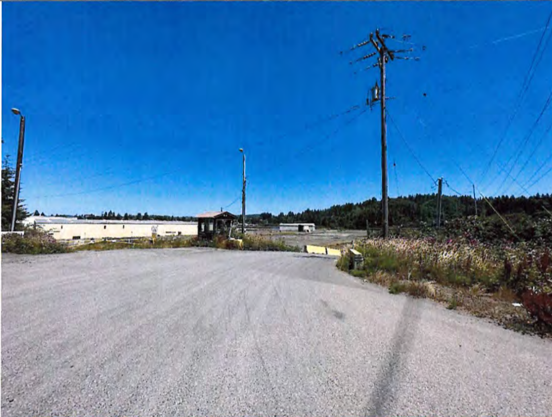
Northeasterly View of Larger Parcel
